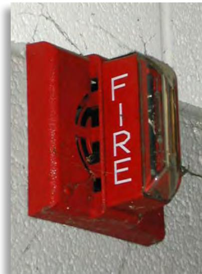
This combination horn strobe notification appliance is part of a fire alarm system that may employ a presignal feature.
