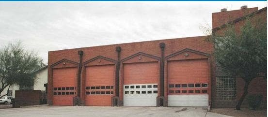
Figure 4.10 — The different colored panels on two of these roll-up doors indicate that they have been damaged in collisions.
