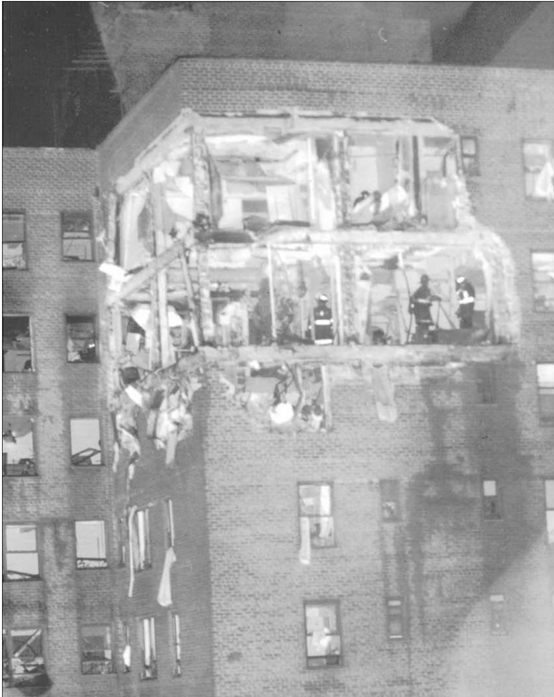
Exterior view of explosion damage on upper floors of 12-story apartment building at 45 East 135th Street, New York City
