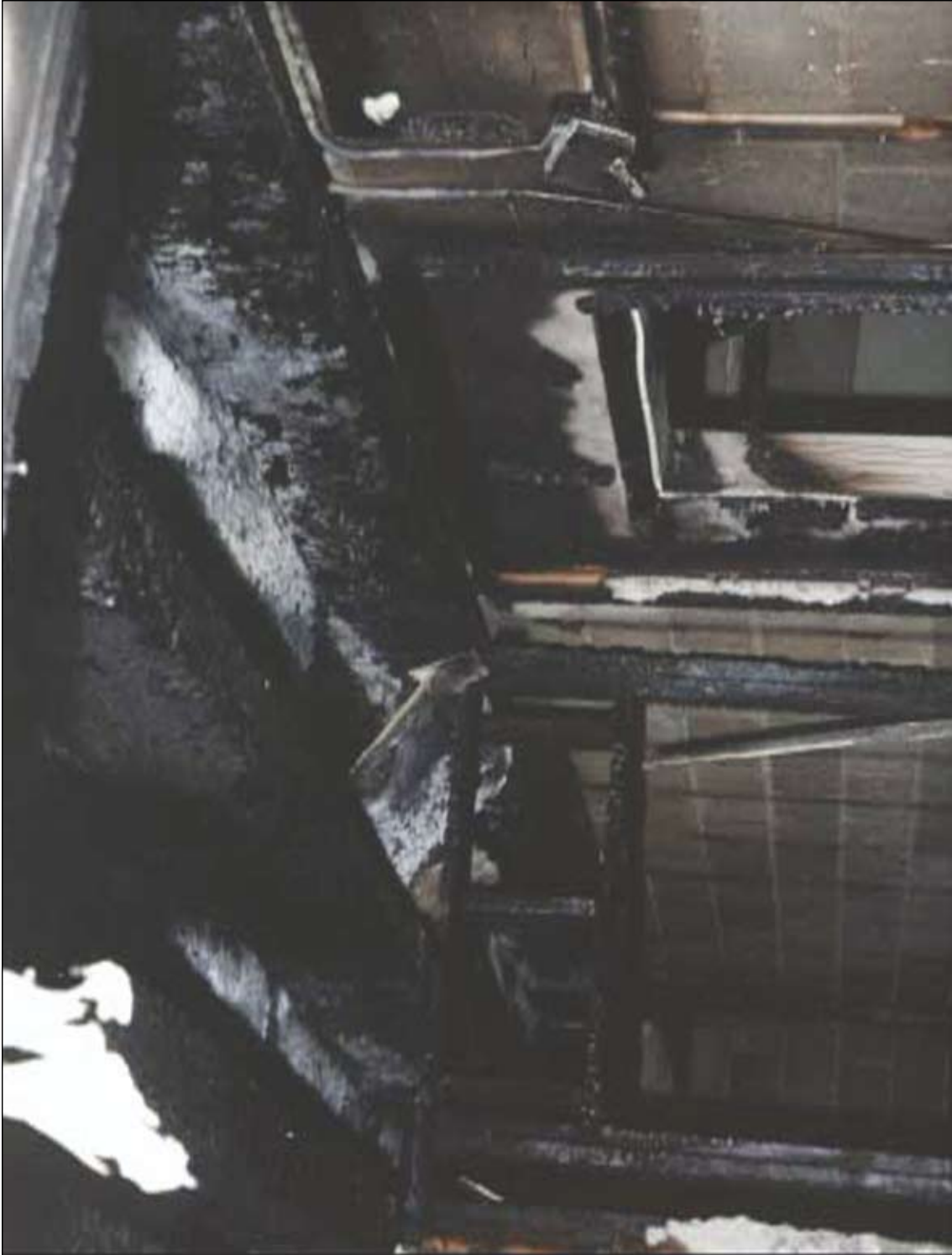
Photo 10. The top of the door frame for the 100 level closet determined to be the point of origin. The open stairway to the 200 level is to the top left off the photograph.
