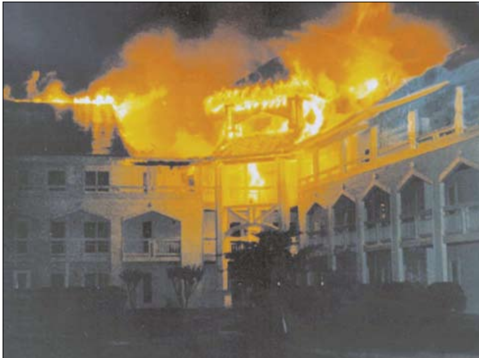
Photo 5. Fire involvement in Sector D (North side) as units were preparing to operate in this sector. The fire was well-established in the attic, third floor walkway, and fourth floor.
