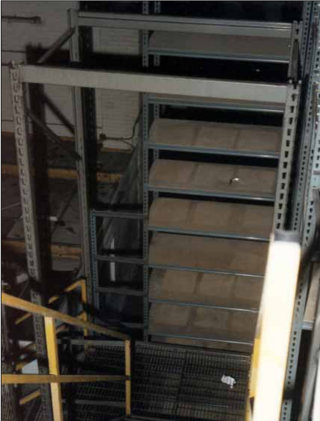
Photo 5. Looking down from the top walkway gives a different perspective to the storage arrangement in the adjacent compartment to the east. Note the solid shelves, unprotected steel racks and typical access stairs.
