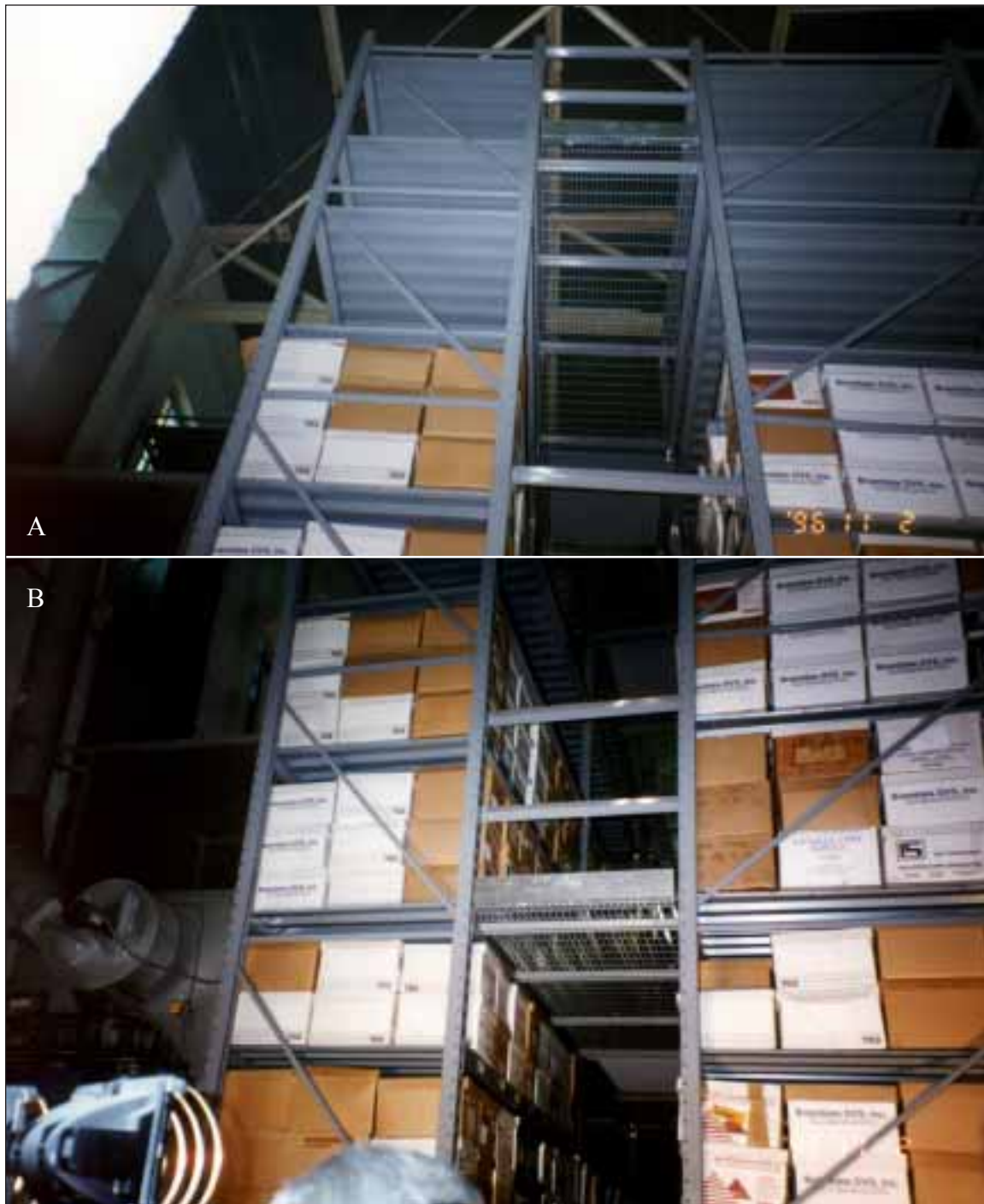
Photo 4. A and B. The shelving and records storage arrangement in the adjacent compartment to the east of the fire compartment. Taken from the floor, the two levels of elevated, grated walkways and the building's roof are depicted.
