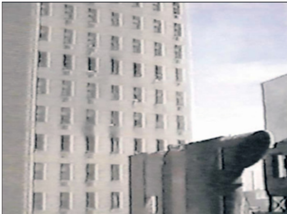
Photo 10. Damage to exposures across Clark Street from the fire building.
