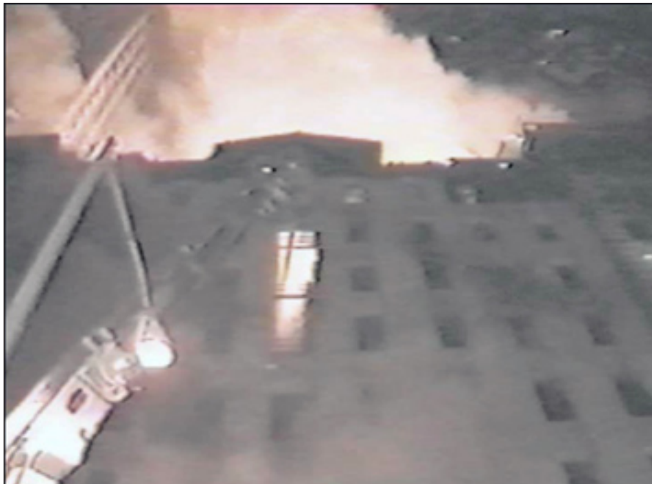
Photo 2. Later conditions on the front of the Clark Building from street level.
