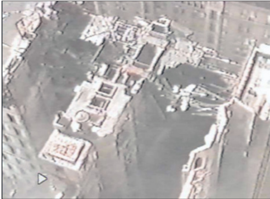
Photo 7. The rear of the Clark Building after the fire. The Tower Building and Grill Building is out of the picture to the right.
