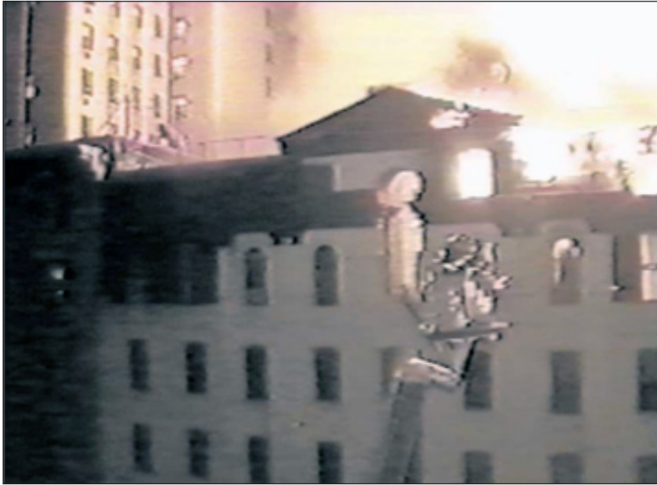
Photo 1. Early conditions on the Clark Street (front) side of the Clark Building with Truck 119 in position to operate its elevated master stream.
